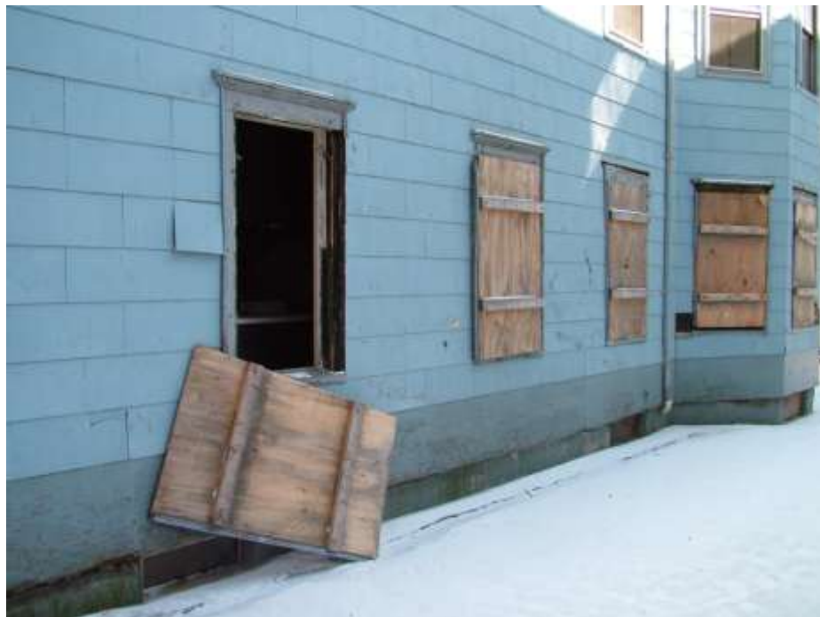
115 Piedmont Street, prior to rehabilitation
